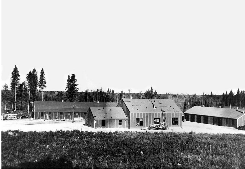
Figure 8.20: Official Canadian Military Photo of Riding Mountain Camp. Northwest facing. Buildings from left to right: barn, garage and workshop, stables. (Courtesy of Parks Canada)
