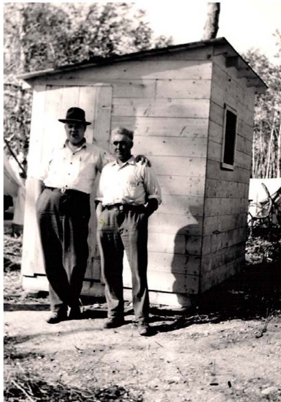
Figure 8.15: Riding Mountain Camp under construction in October 1943. Unknown men standing in front of what was likely a temporary shed used during construction. Note construction worker tents in background. (Courtesy of Pinewood Museum)
