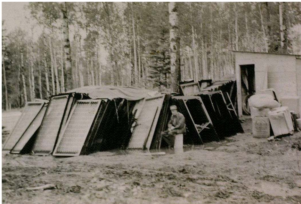
Figure 8.17: Riding Mountain Camp under construction in October 1943. Unknown man with metal bunk bed components prior to assembly. (Courtesy of Pinewood Museum)
