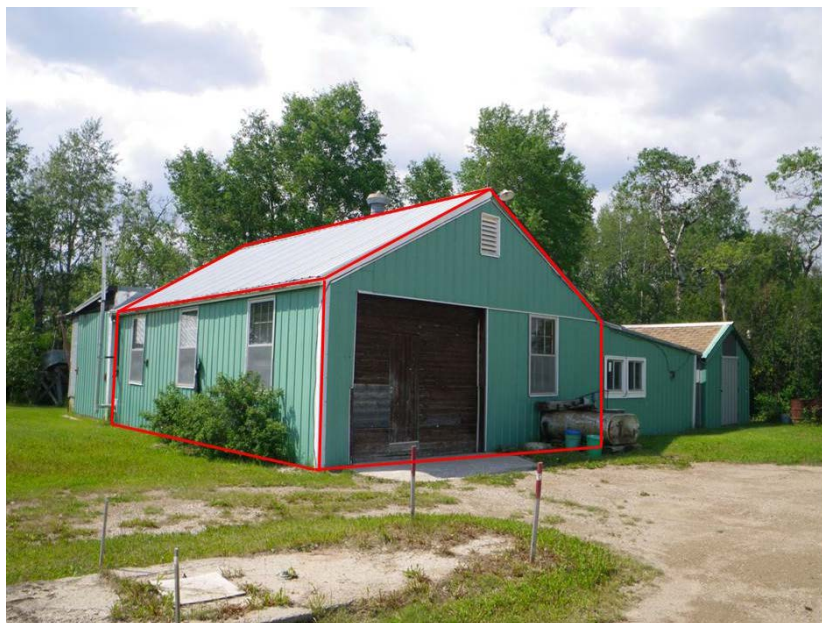
Figure 8.2: The generator building from Riding Mountain Camp, standing today in Strathclair, Manitoba. Note that the building has been expanded. The original structure is outlined with an added thin red line. This building's original foundation is shown in Figure 8.28.
