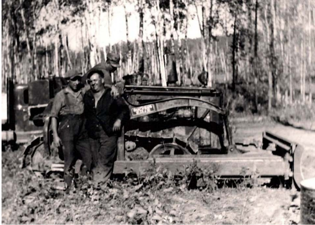
Figure 8.16: Riding Mountain Camp under construction in October 1943. Unknown men with bulldozer used for clearing and leveling ground surface. (Courtesy of Pinewood Museum)
