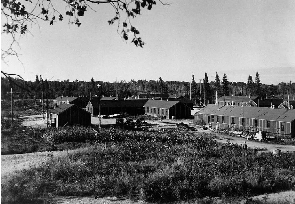
Figure 8.18: Official Canadian Military Photo of Riding Mountain Camp. Southwest facing. The PoW vegetable garden center left. Building on far left is the generator building which stands today in a nearby town. (Courtesy of Parks Canada)
