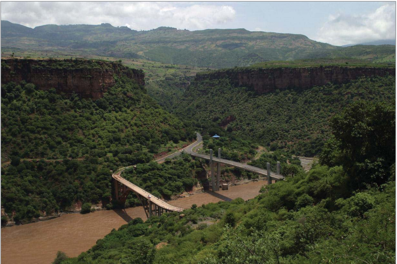
Figure 14. The Blue Nile Gorge at the bridge of the road Addis Ababa – Bahir Dar, 31.08.2012.
