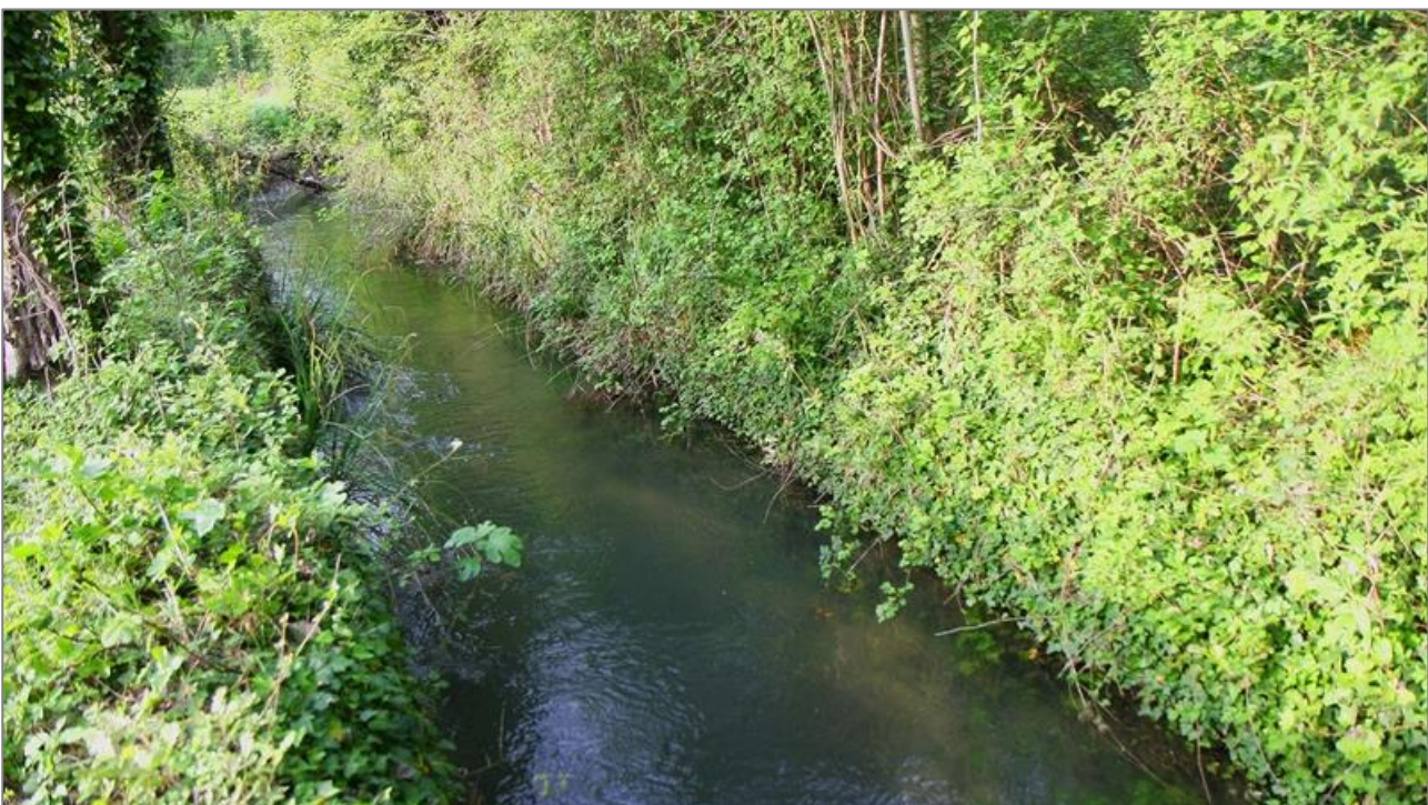
Figure 12. Muratovac canal (Loc. 6)
