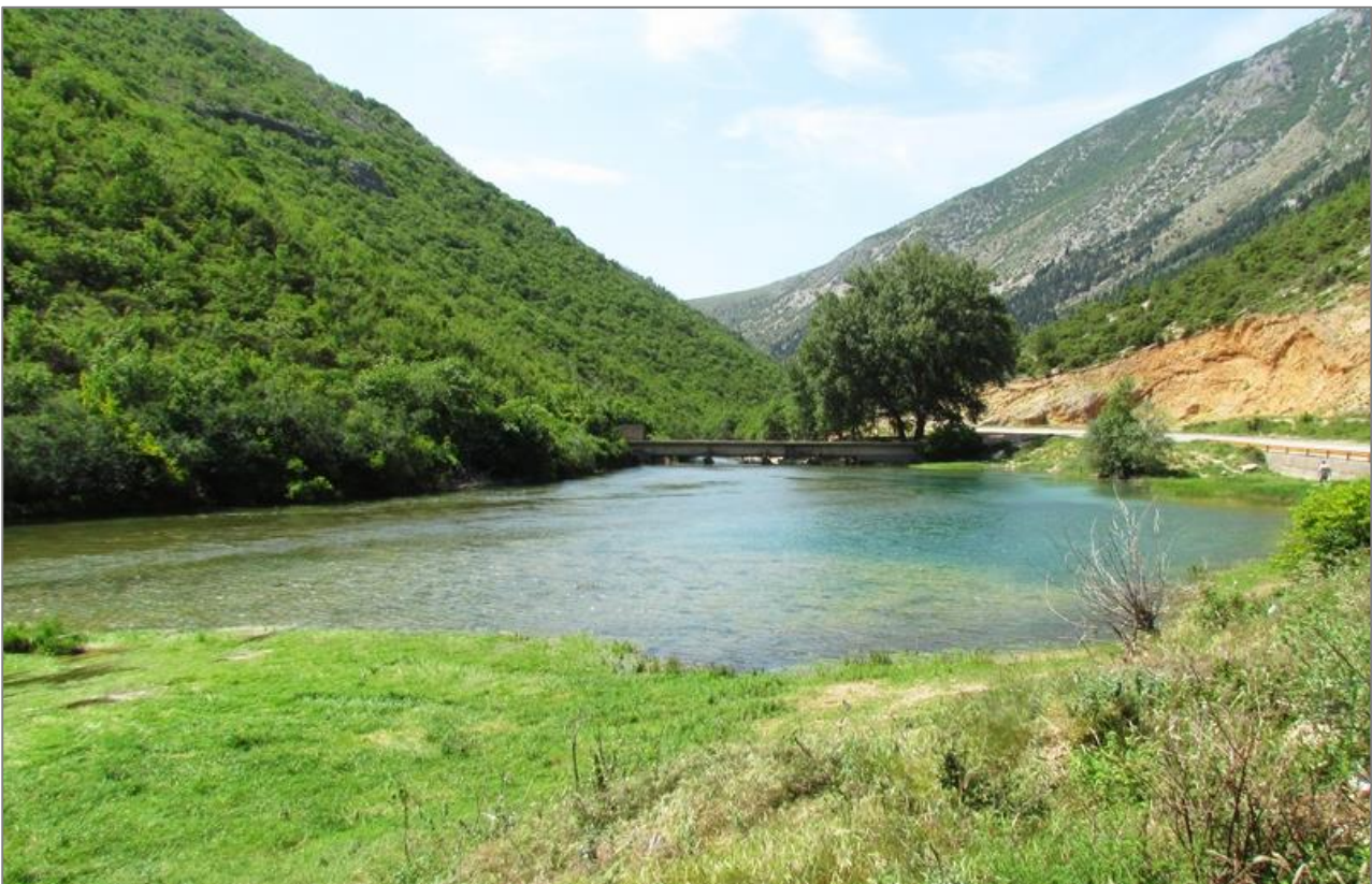
Figure 20. Small dam at Bregava River (Loc. 39)
