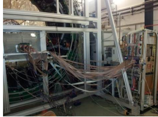
Figure 2.17: Photograph of constructed TOF wall under test
