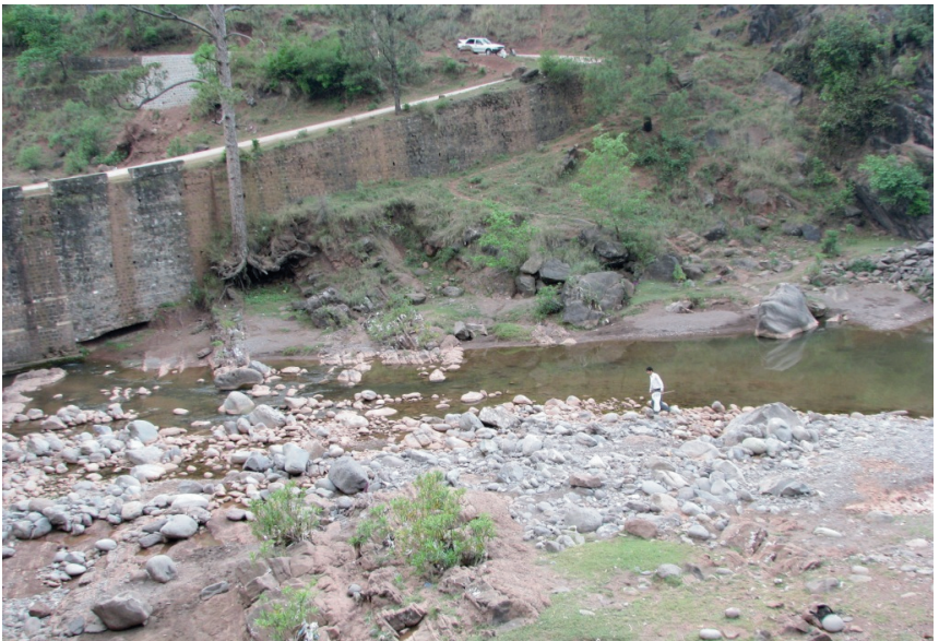
Fig. 14: Angoory bridge spot (East view).
