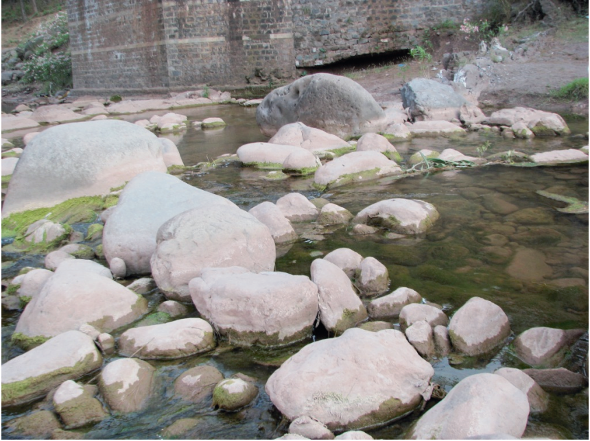
Fig. 13: Angoory bridge spot close up view (East).
