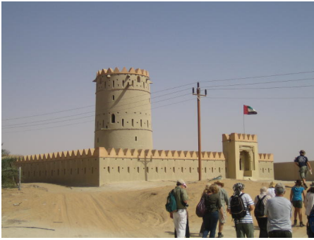
The restored fort at Khannur, Liwa Photograph by Valerie Chalmers
