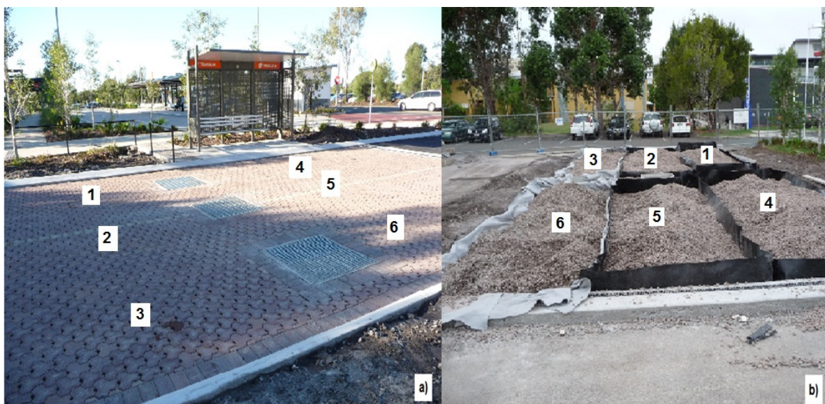
Figure 2. Test locations: (a) after construction; and (b) during construction, showing the six separate treatment sites.
