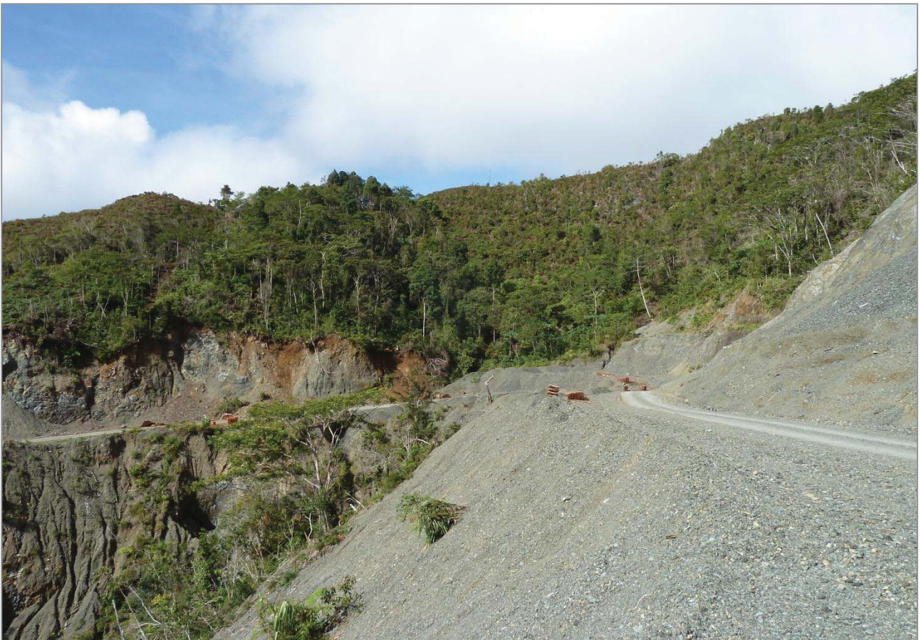
Figure 4c, d. Newly cemented road, cutting the mountain.
