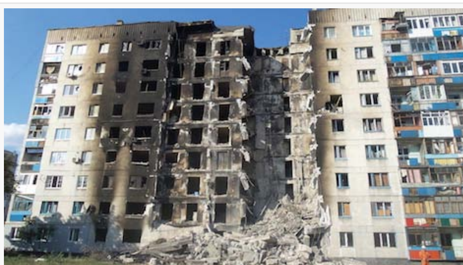
Apartment building in Lysychansk which was destroyed during War in Donbass. (Source: Wikimedia )
