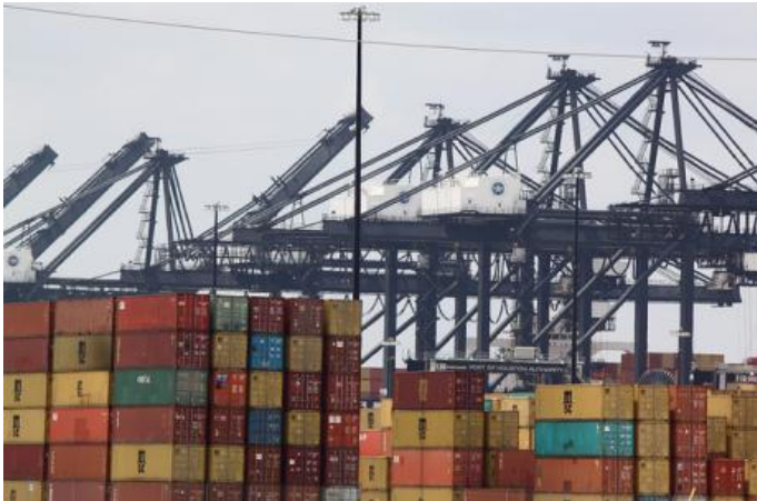
Bayport container terminal, Port of Houston. Flickr/Roy Luck. Some rights reserved.
