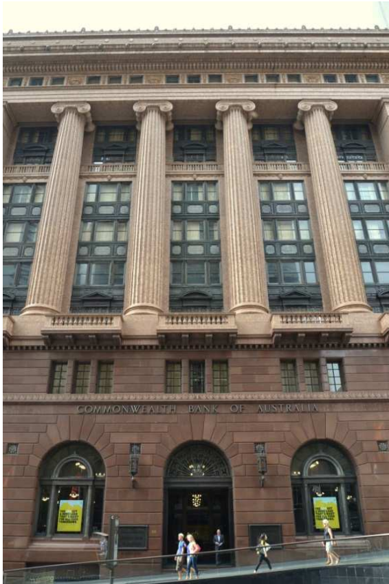
Figure 6: Commonwealth Bank, Martin Place, Sydney
