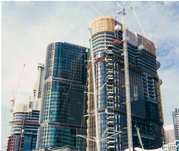
Figure 4: International Towers under construction, October 2015, Barangaroo, Sydney
