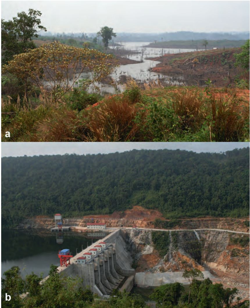
Figure 17. Newly made water reserves at O'Som village (a) and along the road from Koh Kong to there (b). 24.03.2015.
