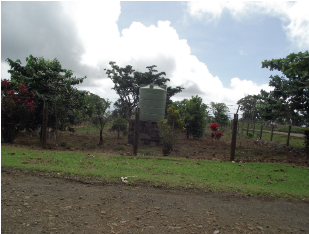
Figure 23. Water tank in Malololelei.
