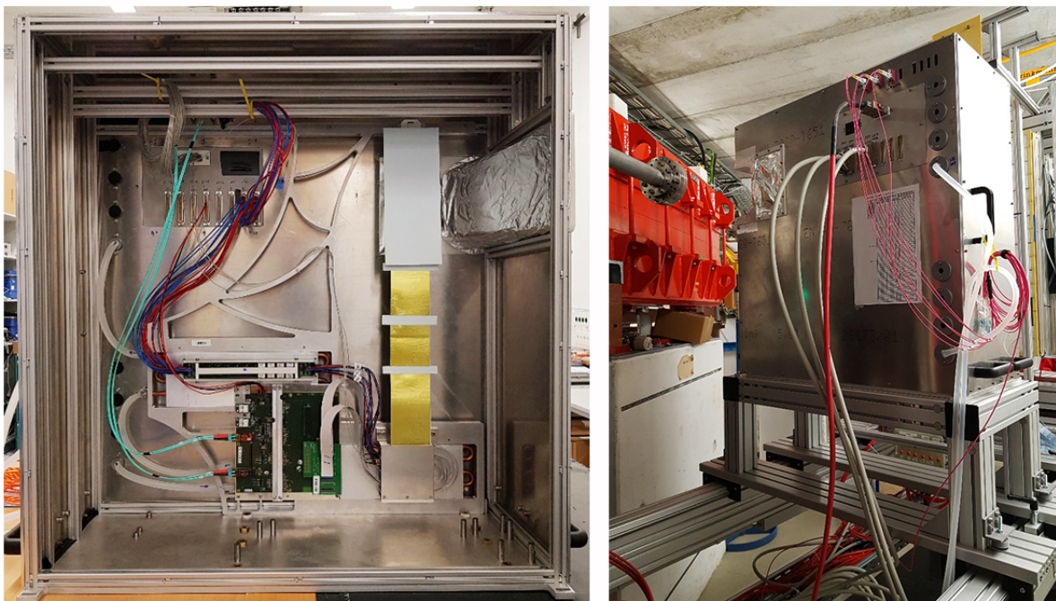
Figure 6.18: Left: Open detector box after full assembly of the main components. Right: Installation of mSTS in the beam line.
