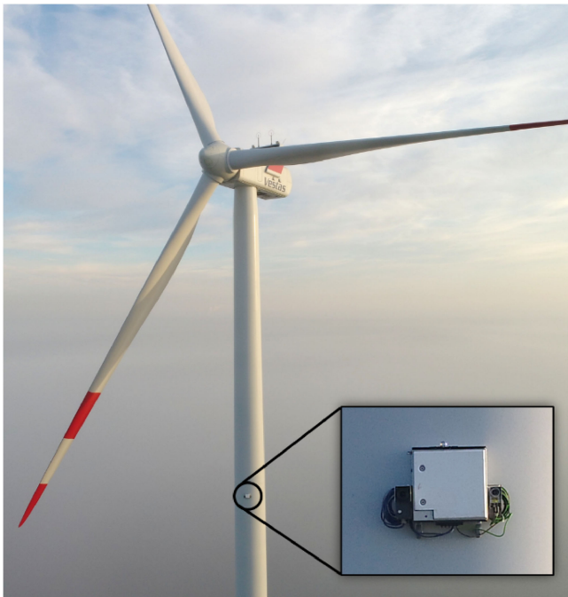
Fig. 10. Illustration of the radar installation at a 2-MW WT at 95 m above the ground. Data were saved on a computer inside the WT tower.
