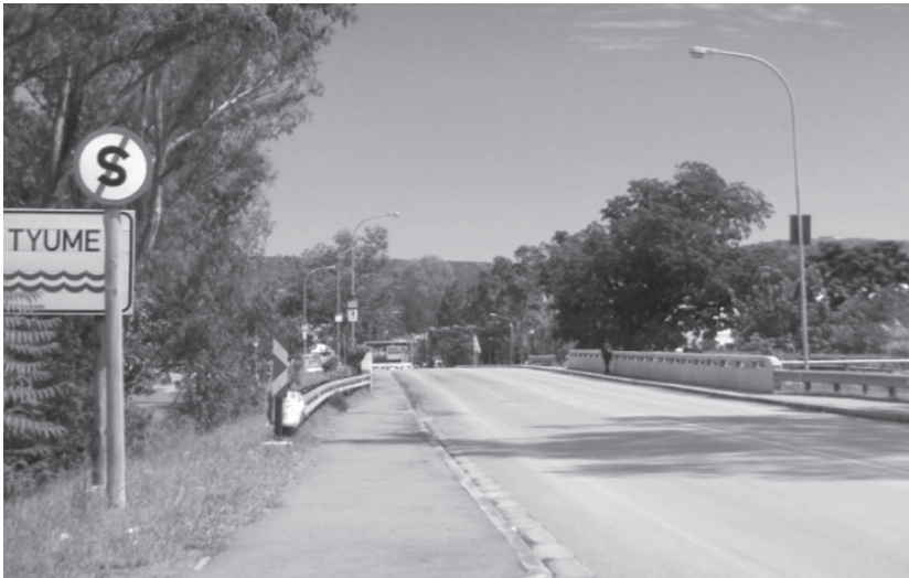
Figure 9.2: The bridge that separates the University of Fort Hare from Alice
