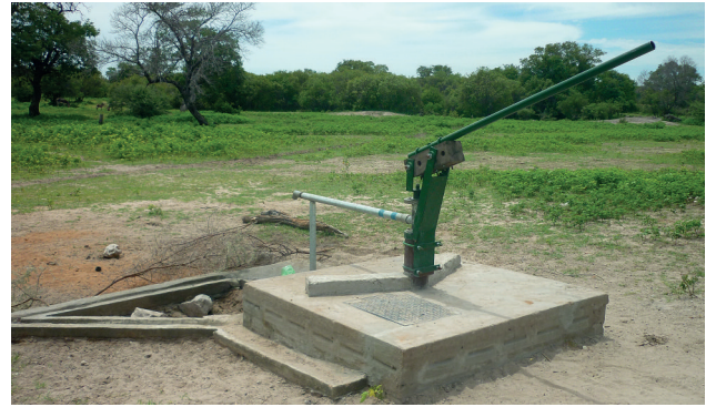
Figure 4: Improved well, that is protected from outside contamination to provide high quality drinking water during the dry season to local and rural communities (Photo: Luetkemeier 2014).
