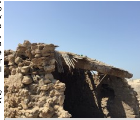
Coral used for construction
