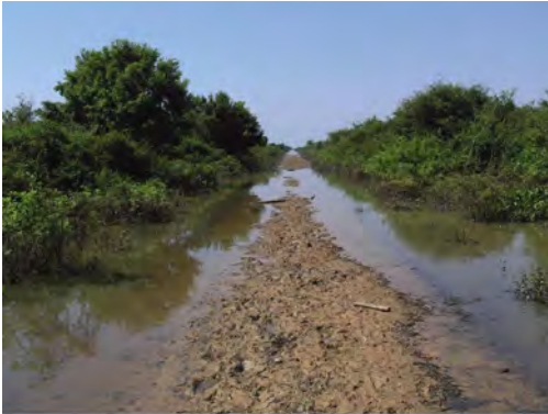
Figure 67. Inundated scrub and a road being released from water at Merchey village (Loc. M), 01.11. 2018.
