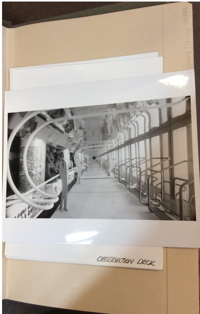
Fig. 14: "Model of the Observation Deck with mirrored ceiling and bench elements being visible." Box 74, Folder 15, WPR.
