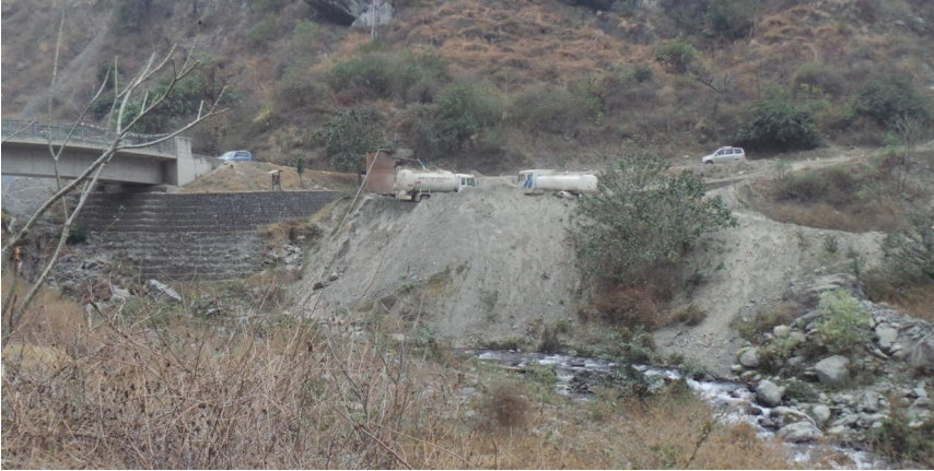
Figure 6. Habitat at site 1 showing the impact of road construction. Larvae of Perissogomphus stevensi , Gomphidae spec and Macromia moorei were collected here.
