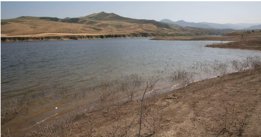
Figure 21. Gazakh district, Abbasbeyli Water Reservoir.
