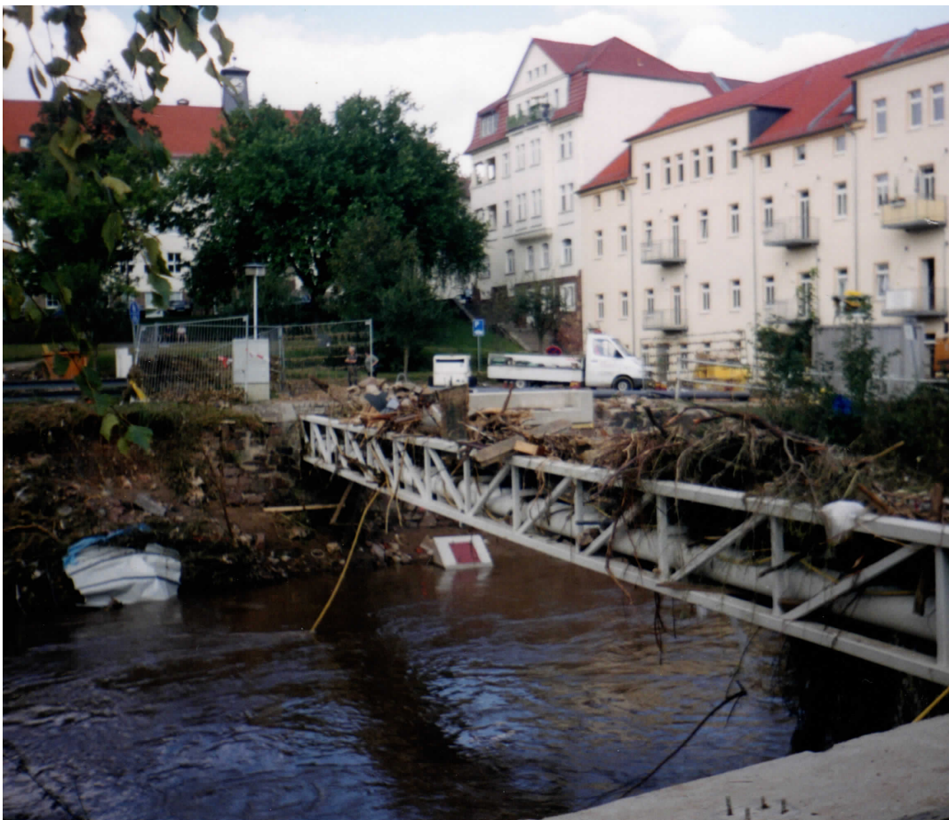
FIGURE 7.1: Bridge in Döbeln (Saxony) damaged by the Vb-cyclone flood in August 2002. Photography taken by Sonja Strini on 23.08.2002 from an opposite perspective than in Figure 6.1.
