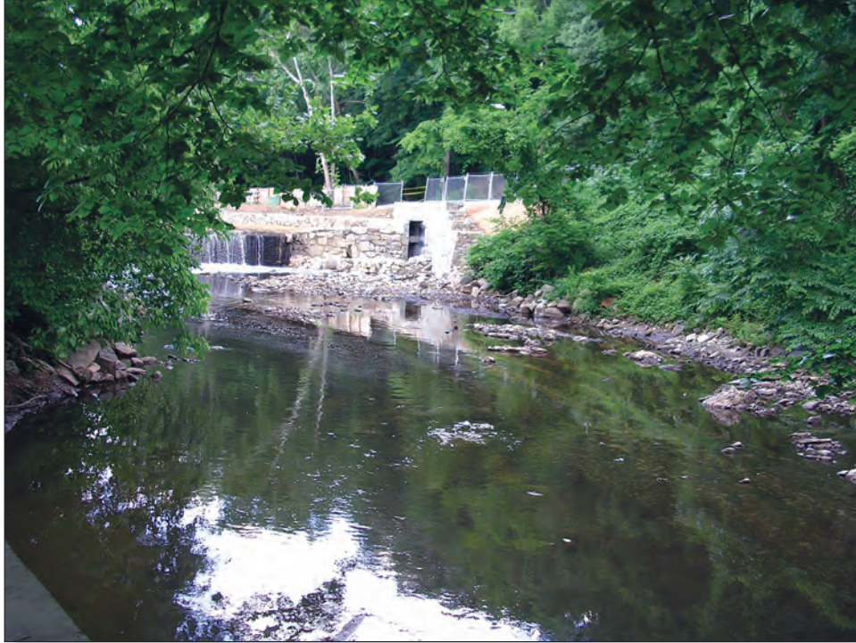
Rock Creek at Peirce Mill, Washington, D.C. (Station 01648016) looking upstream from the millrace at the fish ladder.
