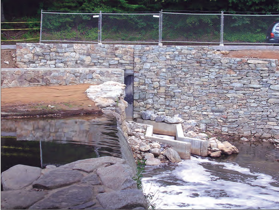
Figure 1. Fish ladder on Rock Creek just upstream from Peirce Mill. [Construction for this ladder was begun after field sampling for this study and was completed in spring 2006.]
