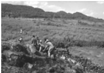
Construction of the buffalo wall with lava rocks
