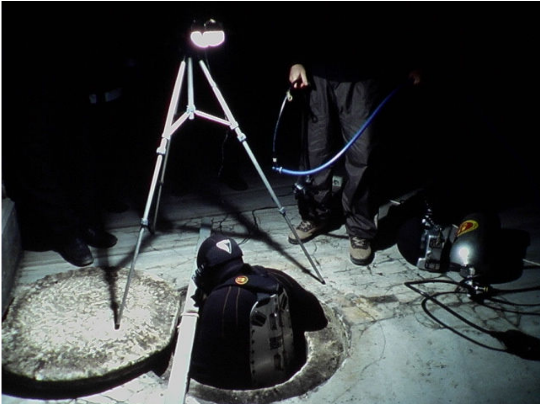
Fig. 6. The hookah system to dive in the well on the southwest of the nave
