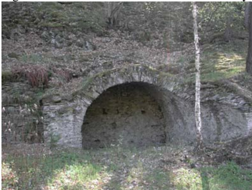
Fig. 6: Closed entrance of a mine from the 19. century. The walls consists of schist.
