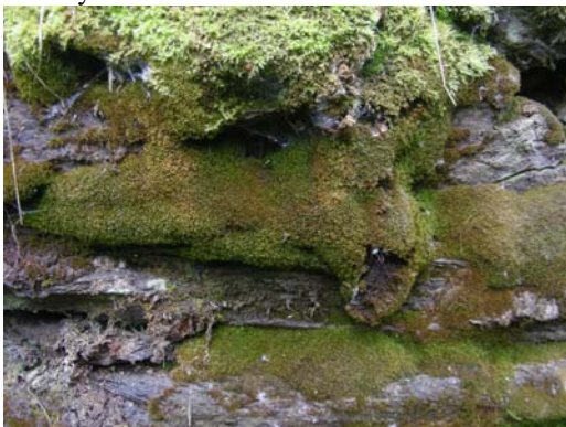
Fig. 8: Wall made from schist in the Gründelbach valley, presumably of a loading ramp.
