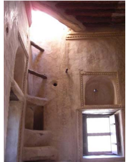
The stair to the viewing level
