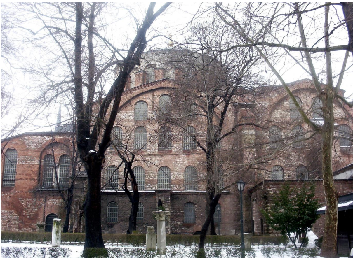
General view. The north flank
