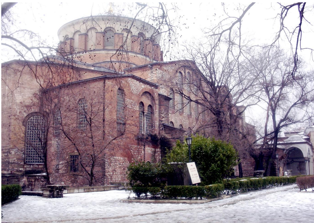
General view –the north flank
