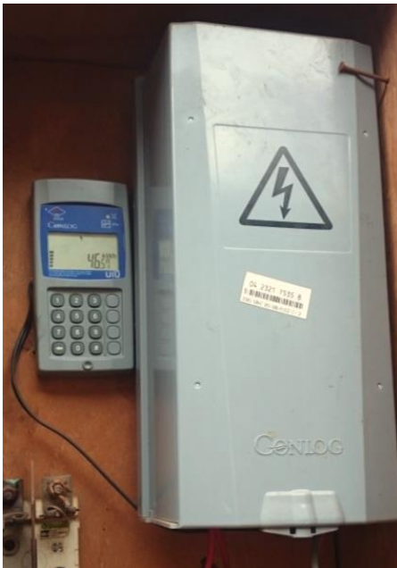
Fig. 7: Pre-paid meter for grid provision
