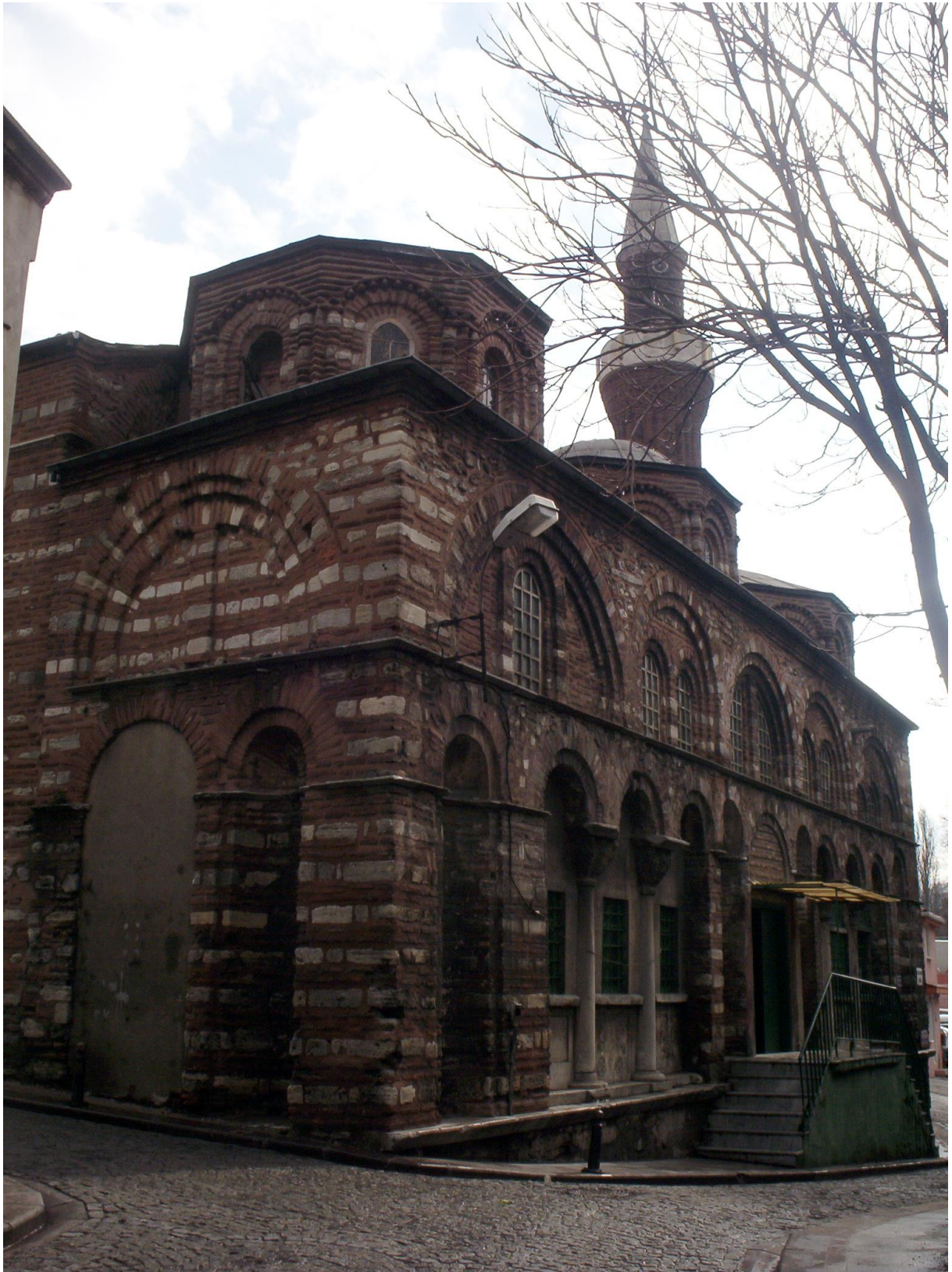
The west façade from the northwest
