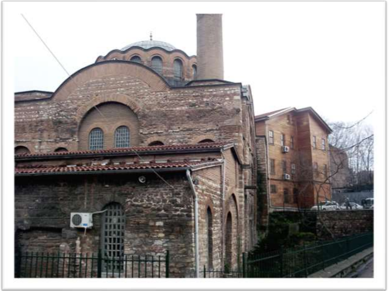
The west façade
