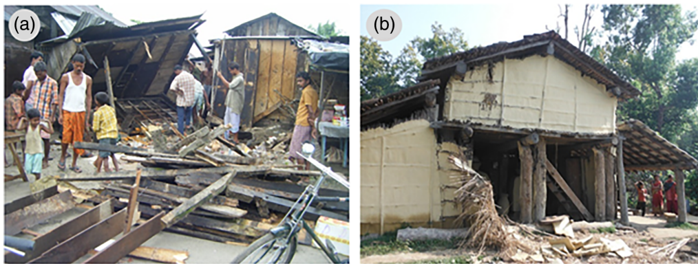
FIGURE 2 Property damage caused by elephants in search for food (a) to a grocery store in Manas at Gadulee Market/Bansbari in May 2009 and (b) to a farmhouse in Bardia at Suryapatuwa in May 2009, where the entire wall has been removed by the elephant
