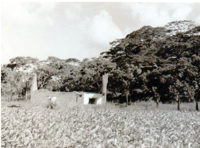
1953: Farm manager's house on Katumba section, Bourton Vale Farm, following a bush fire.
