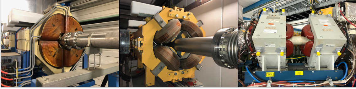
Figure 2.4.: Examples of quadrupole magnets. (left: quadrupole doublet from the transfer channel UNILAC to SIS18, centre: quadrupole doublet from high energy beam line, right: quadrupole doublet from Crying local injector line)
