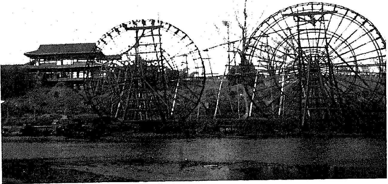
1. CHINESE WATER WHEELS MADE OF BAMBOO
