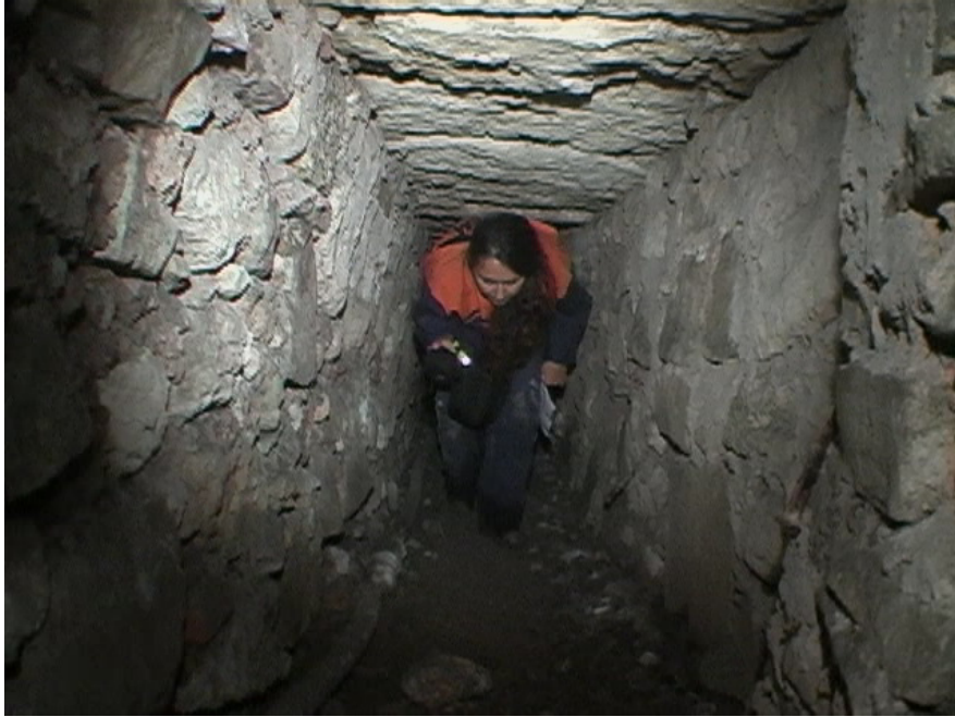
Fig. 2. The tunnels connected to the vaulted passage
