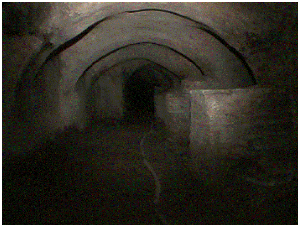
Fig. 1. The vaulted passage under the inner narthex
