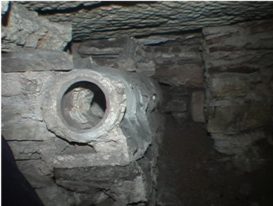
Fig. 3. The water pipe that seems to head towards the atrium
